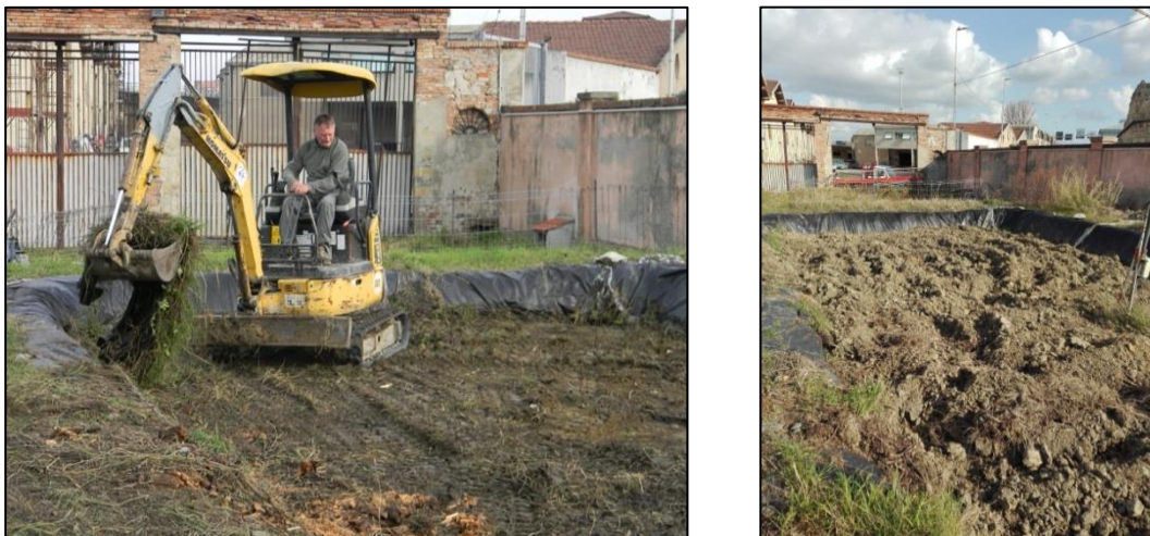
Figure 2. Landfarming process with little excavator
